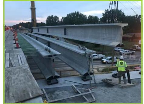
Beams being set for the bridge deck for the I-70 widening project over Springfield-Xenia Rd. (photo courtesy of Michelle Porr)
