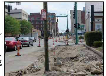
Fountain Ave. streetscape (2013)
